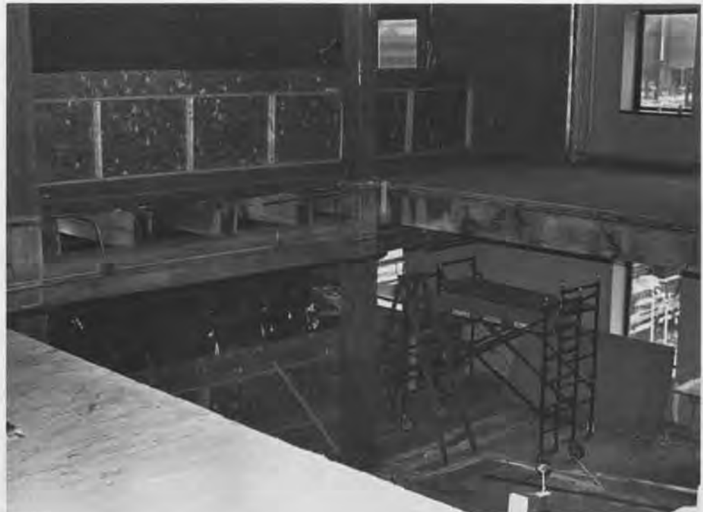
Bay 4 on floors five and six readied for a central staircase.
