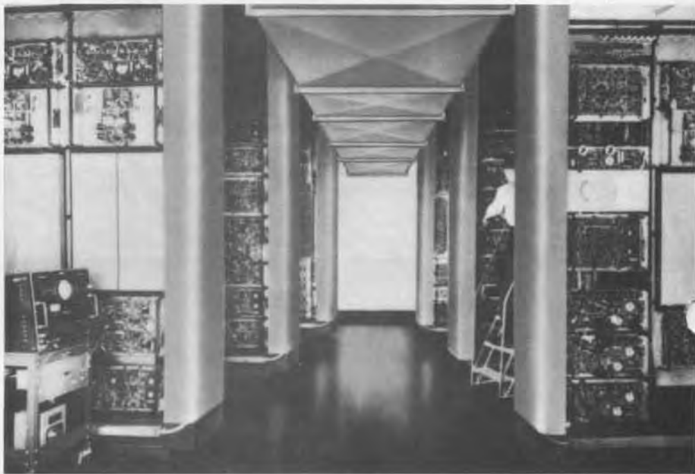
Entrance into the Museum puts the visitor in Whirlwind's arithmetic units, which occupied a whole room in the Barta Building at MIT. The 16 bit word length, extending 32 feet, was partially determined by the width of the room.
