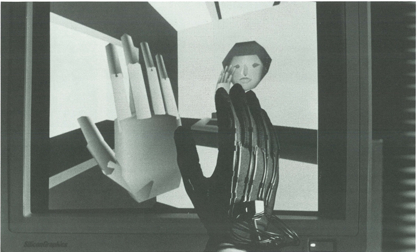
A special sensor-equipped glove permits manipulation of simulated objects in a computer generated world of "virtual reality."
