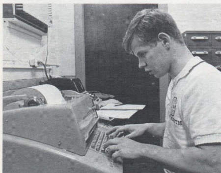
Flexowriters were used to punch the paper tape for the input of data for many of the first computers. These machines and their antecedents were cheaper, stored upper and lower case, and had a better human interface than the punched-card machines. They led directly into the development of computers with keyboard input.
