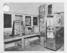
Electrical Testing. Core drivers helped in electrical core testing. The cores, which were temperature sensitive, were tested at a uniform 25 C. The temperature was controlled by core handlers in temperature-regulated boxes or air-conditioned rooms.
