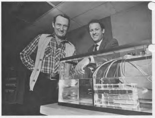
Seymour Cray and John Rollwagon, President and Chairman of Cray Research, standnext to a prototype of the CRAY-2. To keep i components cool, the entire CPU will be immersed in inert fluorocarbon, the substance used for artificial blood.
