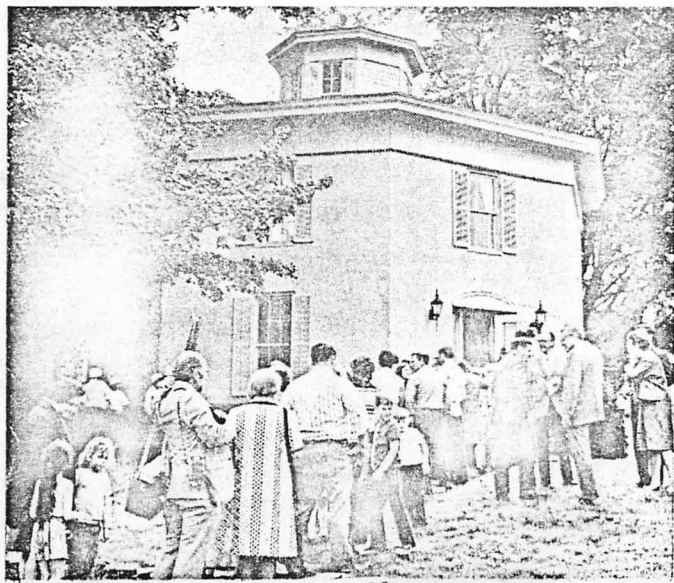
Rare octagonal house in upstate New York is site of Glad- ding Corporation's International Sport Fishing Museum.
